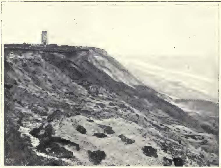
A landslip on the Norfolk coast.
